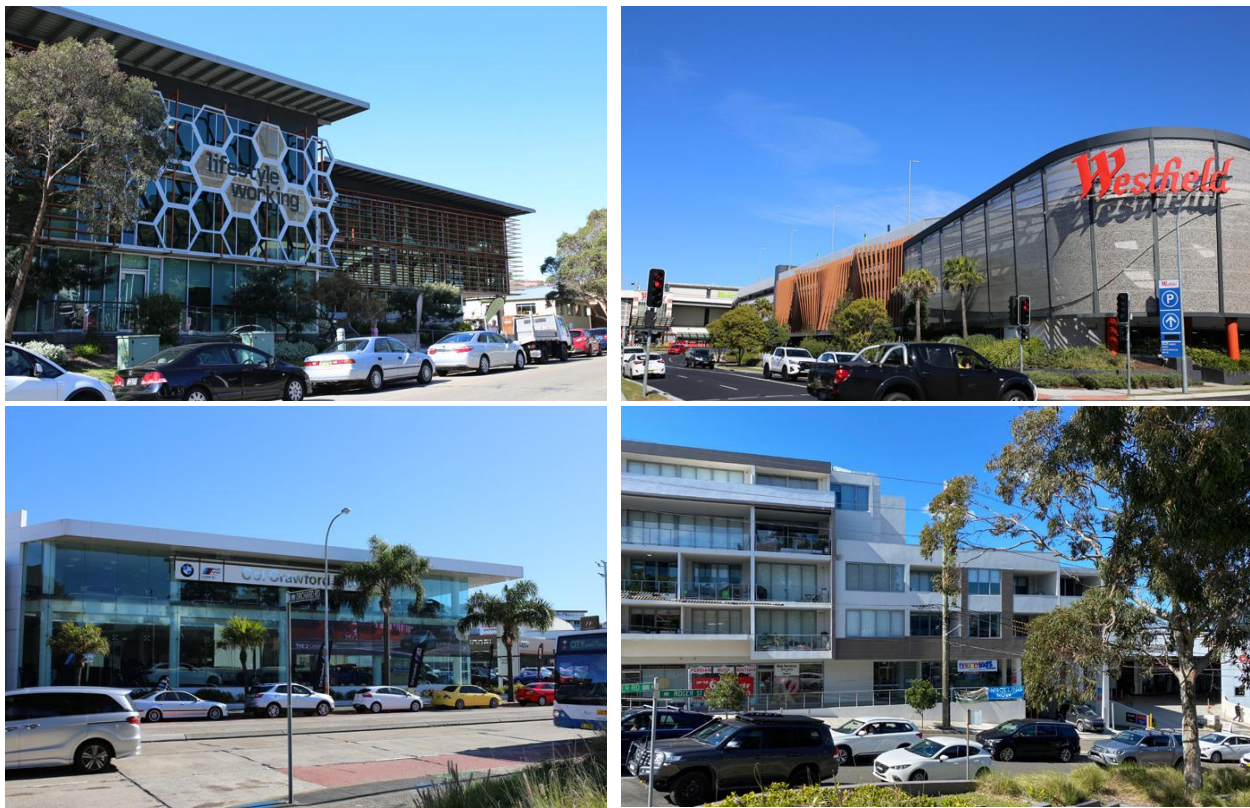
Figure 2 Existing built form
